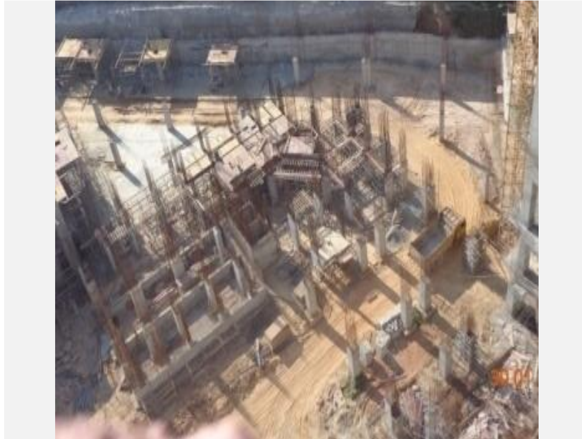
TOWER L : Lower Basement Slab Shuttering Works in Progress
